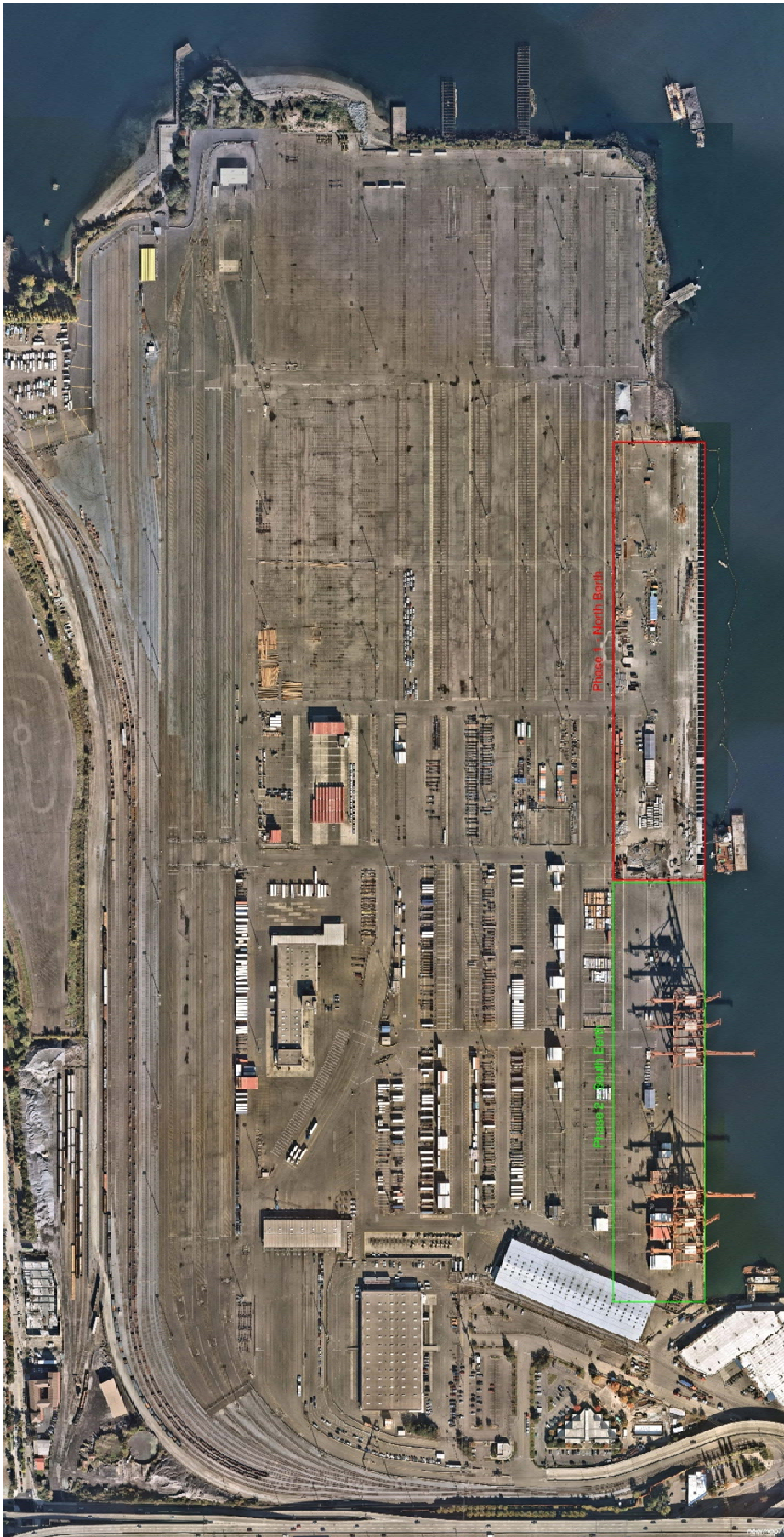
T5 Wharf Phases – Phase 1 North Berth (red) and Phase 2 South Berth (green)
